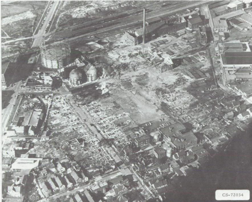
Figure IX-1. - Liquid-natural-gas storage tank failure. (Photograph by Cleveland Plain Dealer.)
